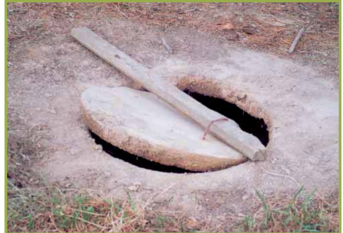
Example of a well constructed offal pit
