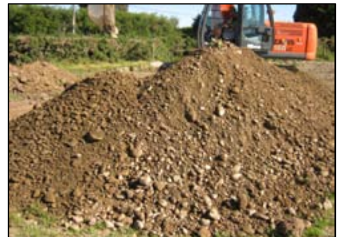
Photo 6: Gravel removed from Test Pit.
