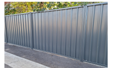
1.8M HIGH AU PREFINISHED COLOURED STEEL PANEL IN 'MONUMENT' COLOUR.
