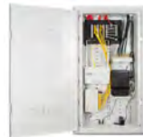
Patch Panel Fibre Connection
