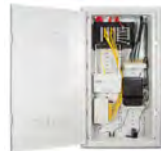
Patch Panel Fibre Connection
