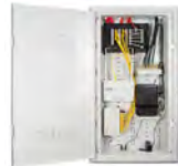
Patch Panel Fibre Connection
