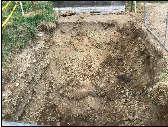
Photo 1: Area 1: Waste pit after removal
