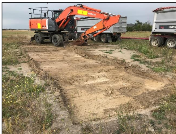
Photo 5: Area 7: Burn pile after removal
