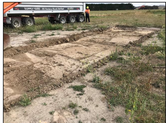
Photo 6: Area 7: Burn pile after removal
