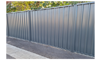
1.8M HIGH AU PREFINISHED COLOURED STEEL PANEL IN 'THUNDER CLOUD' COLOUR.
